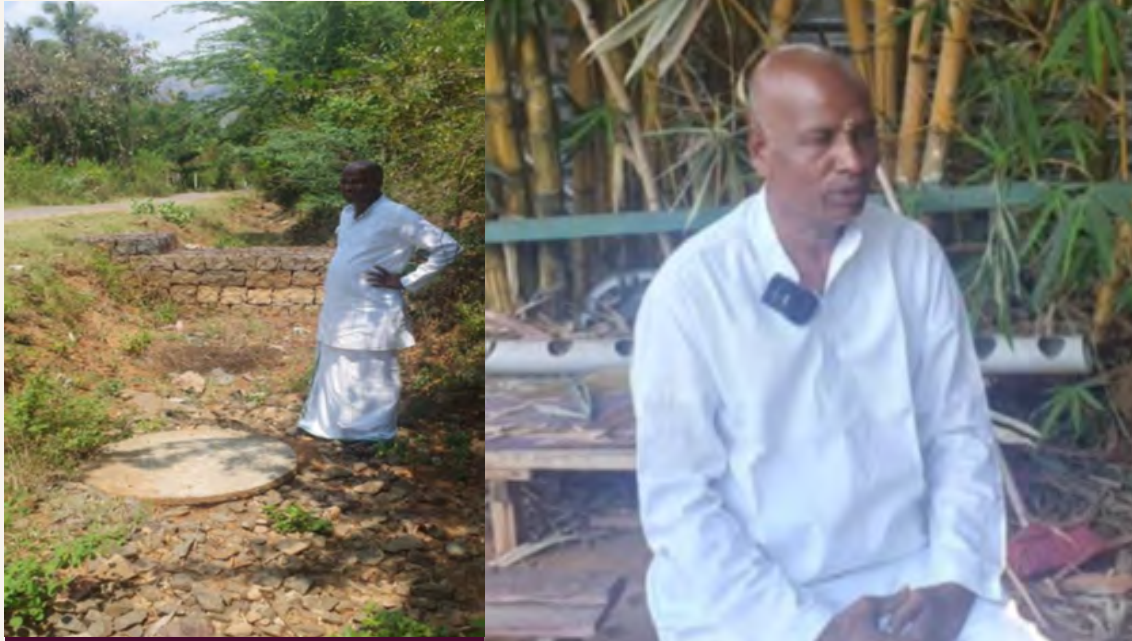
The recharge well stored water and the check dam controlled the flow of water
