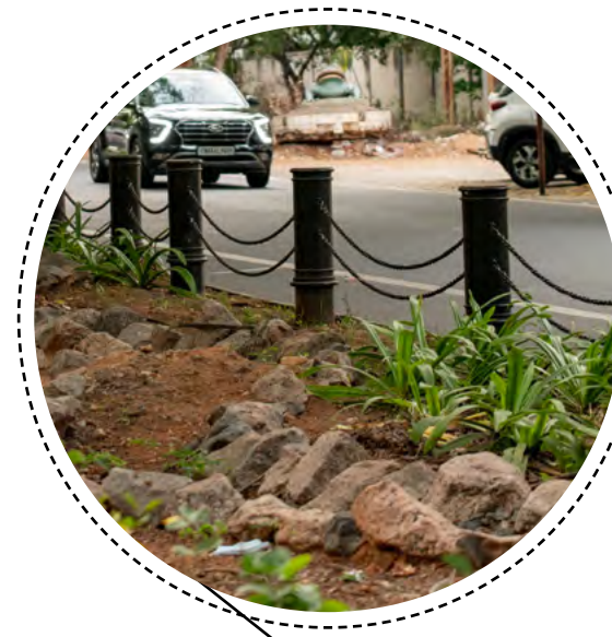
Stormwater swale within the landscape zone
